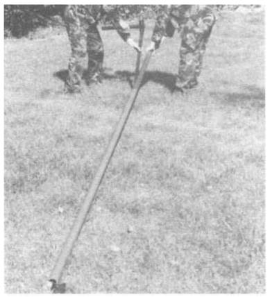
Marking out the guy radius, using 3 mast sections.
