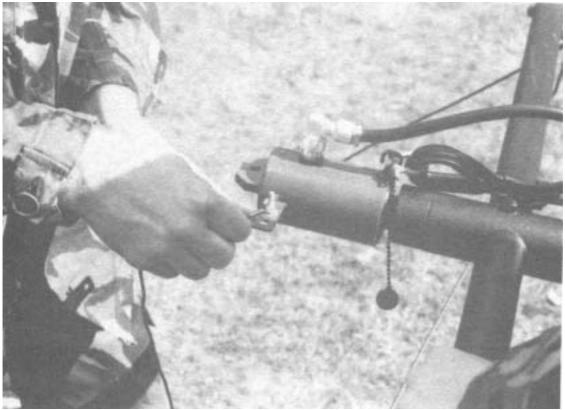
Connecting the antenna elements to the balun transformer.
